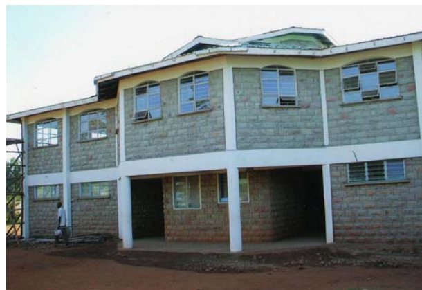
DEC – second phase building completed
